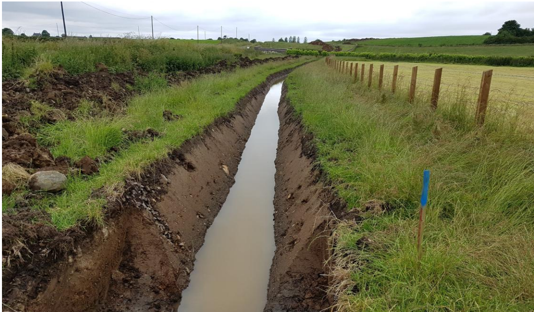
Plate 4-1 - Example of cut-off ditch
