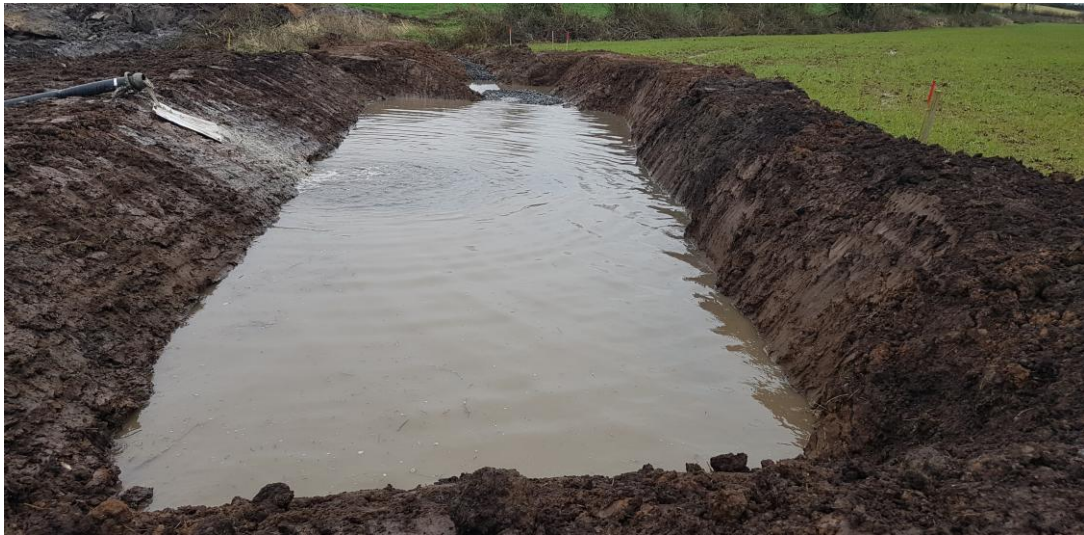
Plate 4-5 - Typical temporary settlement pond / lagoon
