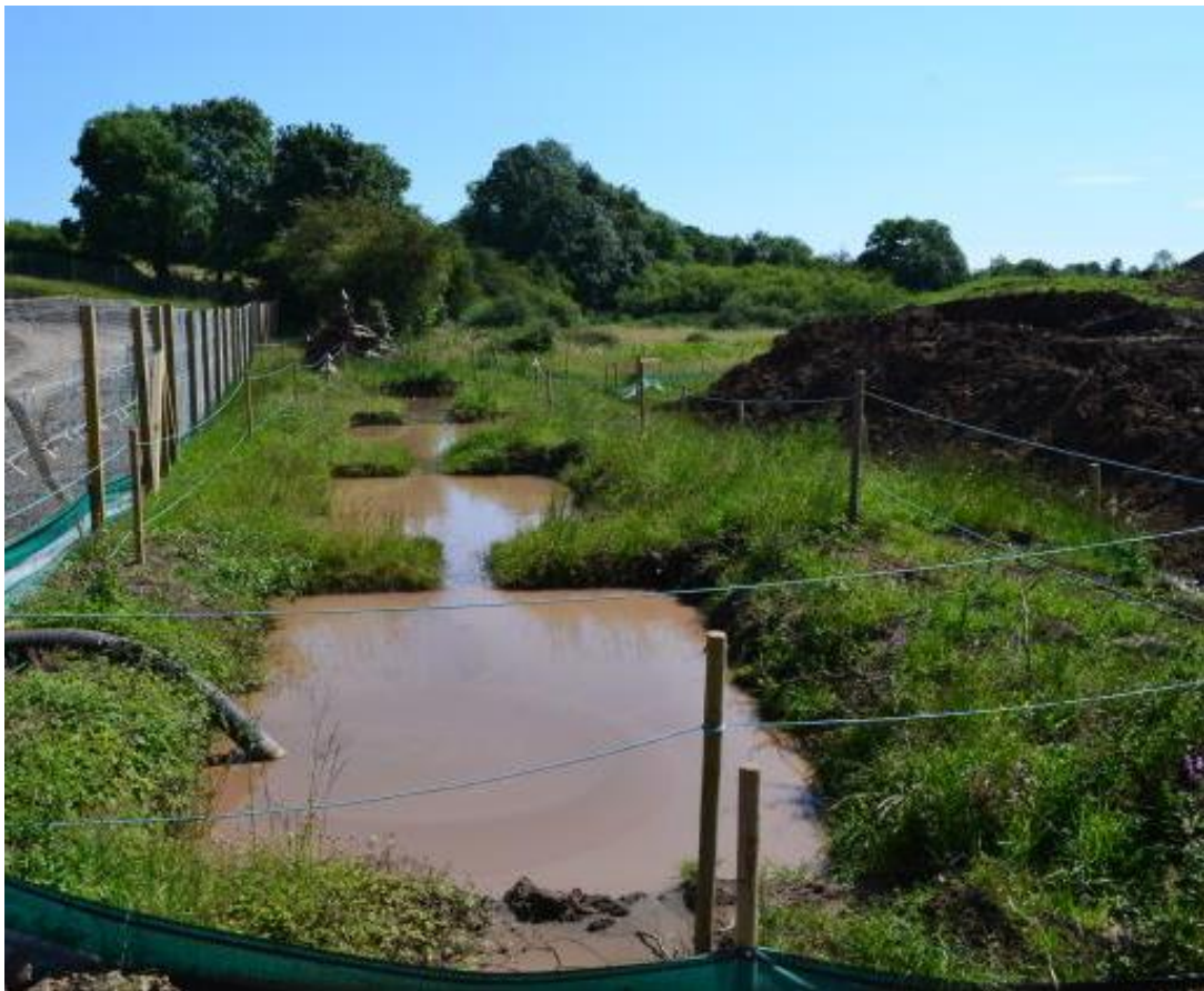
Plate 4-3 - Typical temporary settlement pond / lagoon
