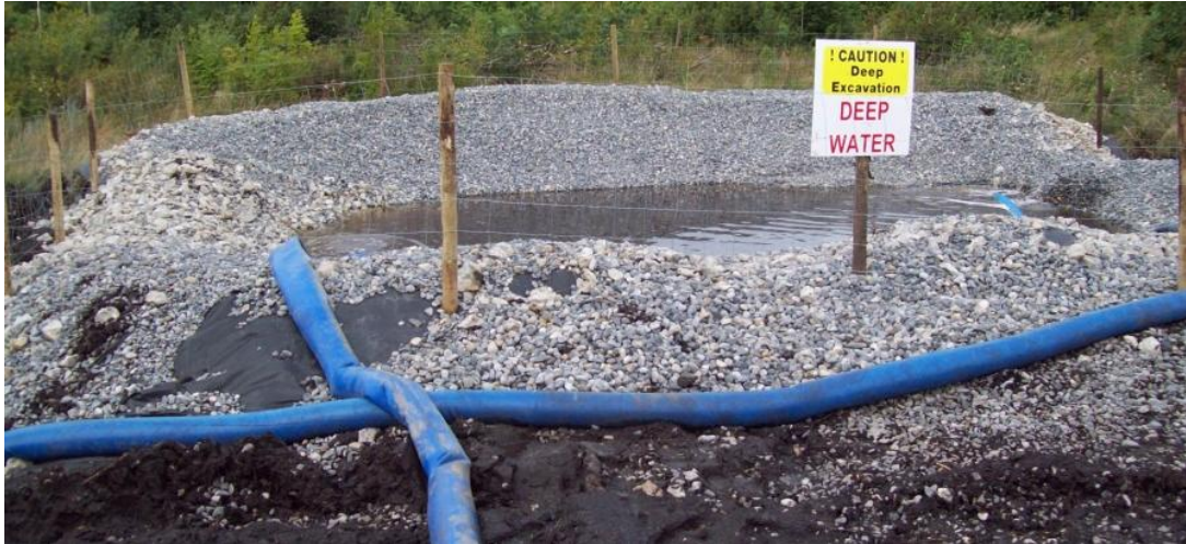
Plate 4-4 - Typical temporary settlement pond / lagoon
